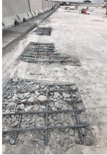
Figure 21: Low Concrete Cover and Rebar Corrosion after Asphalt and Waterproofing Removal
