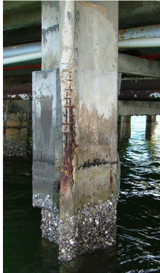
Figure 4: Localised Corrosion at Tidal/Splash Zone of Marine Piles
