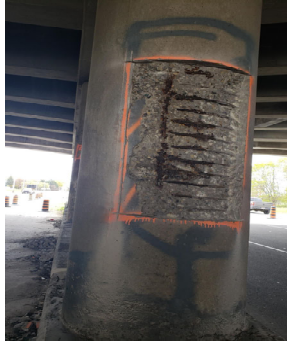
Figure 16: Pier Column Corrosion, Corrosion Protection and CFRP Strengthening for the Pier Columns
