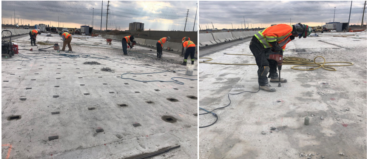
Figure 22: Chipping Pockets in Low Cover Area and Drilling holes for Anodes
